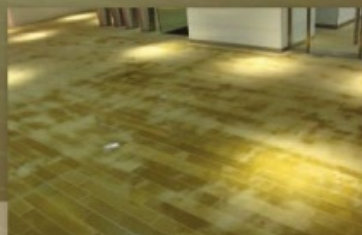
Stone floor immediately after treatment
